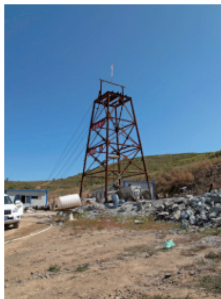
Figure 4 – New Vertical Shaft #8
