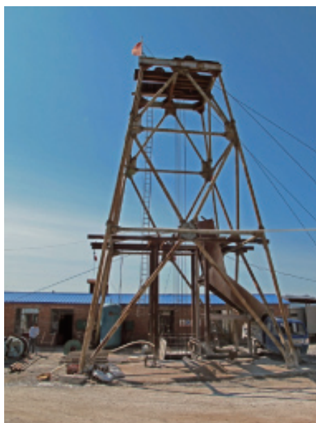
Figure 3 – New Vertical Shaft #2
